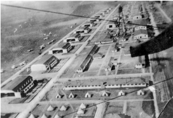
Aerial view of the hangars of Benbrook Field (from the Benbrook TX Public Library, via Corky Baird).
